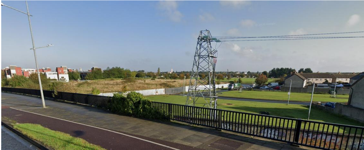
Figure 2-3 View of the site showing the existing network of Pylon and Overhead lines (Source: Google maps).
